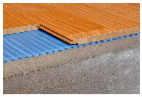
Determination of alternate vertical movements on the structure of ProVent underlay and joints of the parquet/laminate floor.
